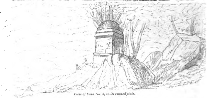
View of Casa No. 4, in its ruined state.
