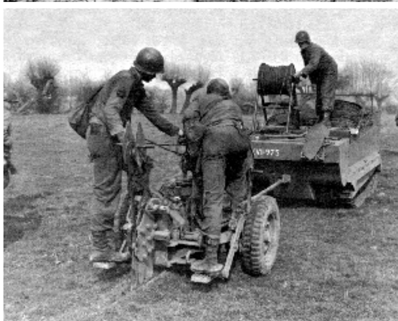
The work of a World War II signalman could take him to new heights—as in the case of this lineman atop a telephone pole—or to new depths, as demonstrated by these men burying spiral-4 cable near the Rhine.
