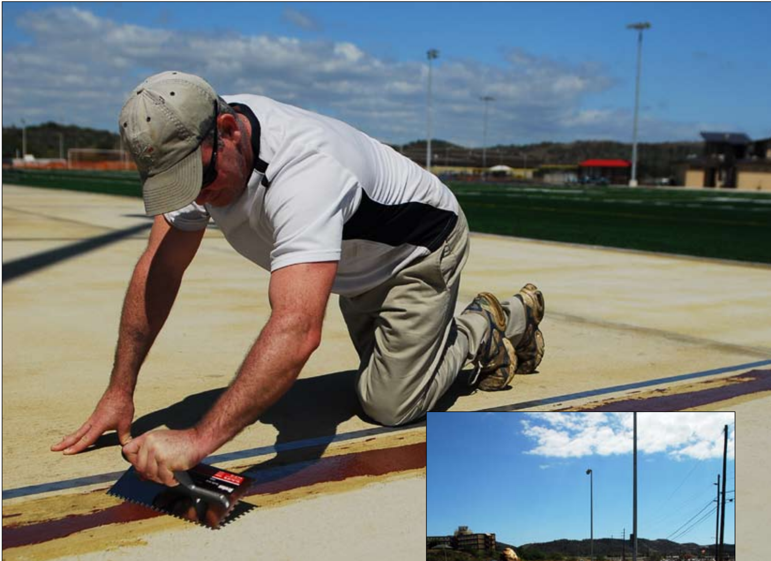
(Above) A contractor trowels gap filler as part of preparations for the track at the Cooper Sports Complex prior to “resurfacing”. It will re-open April 1 and will mark the end of the MWR project and completion of the sports complex. (Right) A contractor spreads the first layer of rubber on the track at the Cooper Sports Complex.
