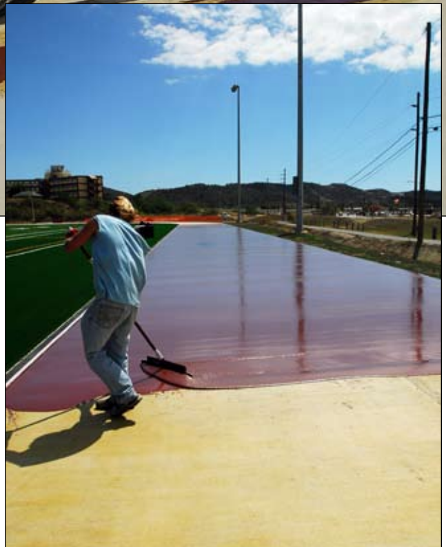
(Above) A contractor trowels gap filler as part of preparations for the track at the Cooper Sports Complex prior to “resurfacing”. It will re-open April 1 and will mark the end of the MWR project and completion of the sports complex. (Right) A contractor spreads the first layer of rubber on the track at the Cooper Sports Complex.
