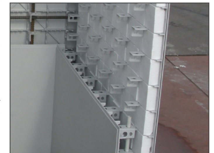
Polystyrene Insulation Insert
