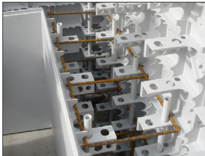
Trench Mesh Used to Create a Wider Wall
