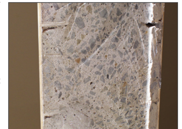
Finished Wall Cross Section
