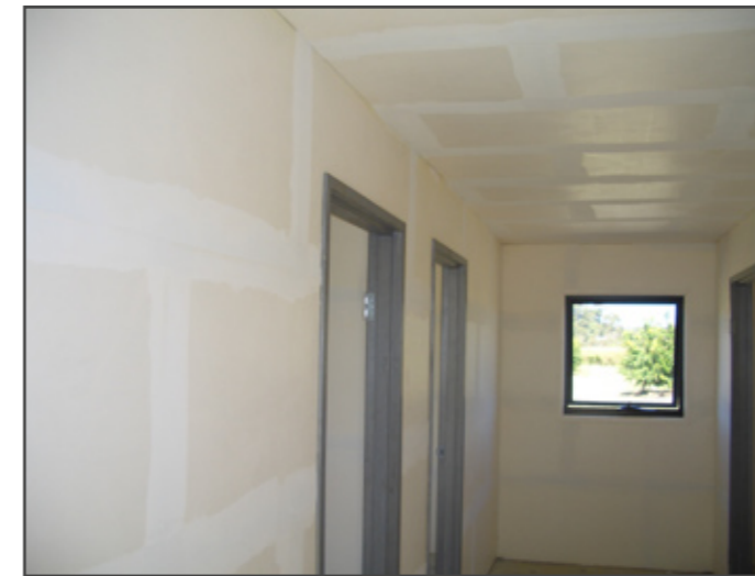
Flushed Walls & Ceilings
