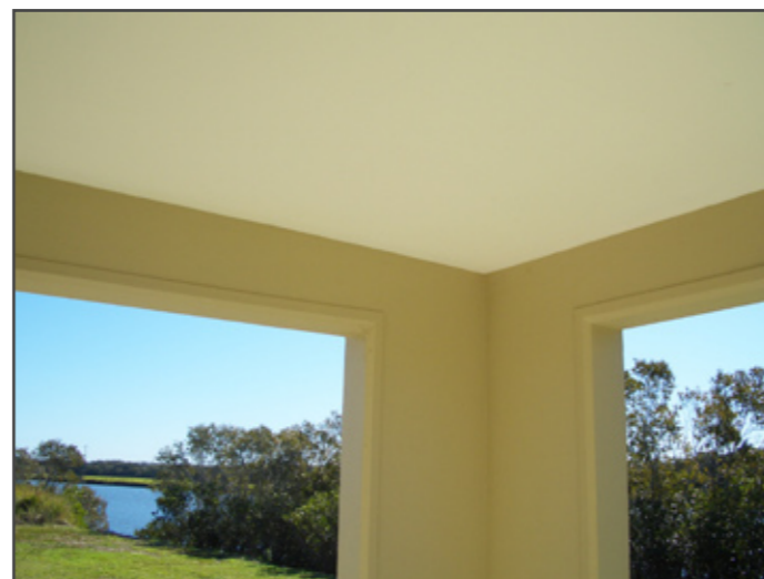
Finished Wall and Ceiling Surfaces
