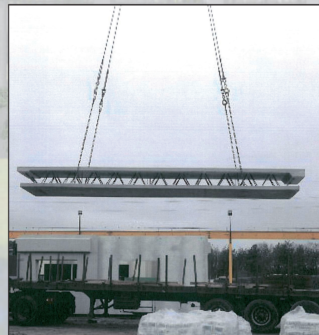
20m 1 span, 0.7m thick concrete double floor
