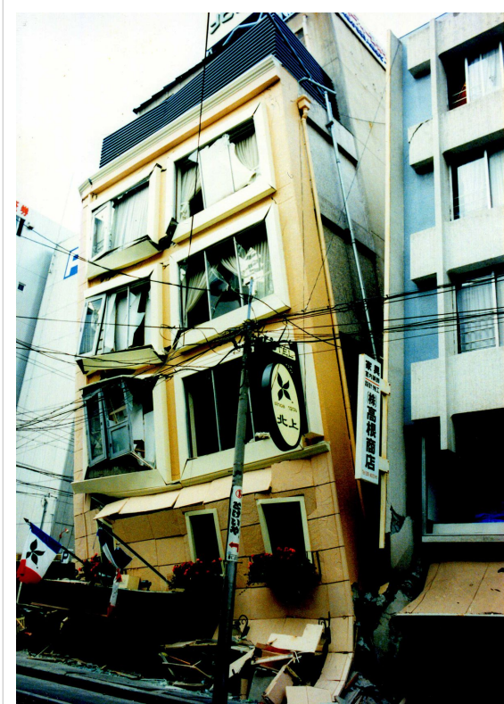
Damaged buildings from the Hanshin-Awaji earthquake of 1995 in Chuo-ku Kobe city.
