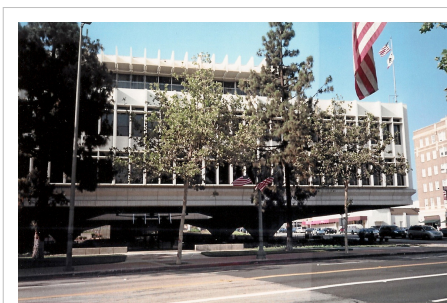
Seismically retrofitted Municipal Services Building in Glendale, CA
