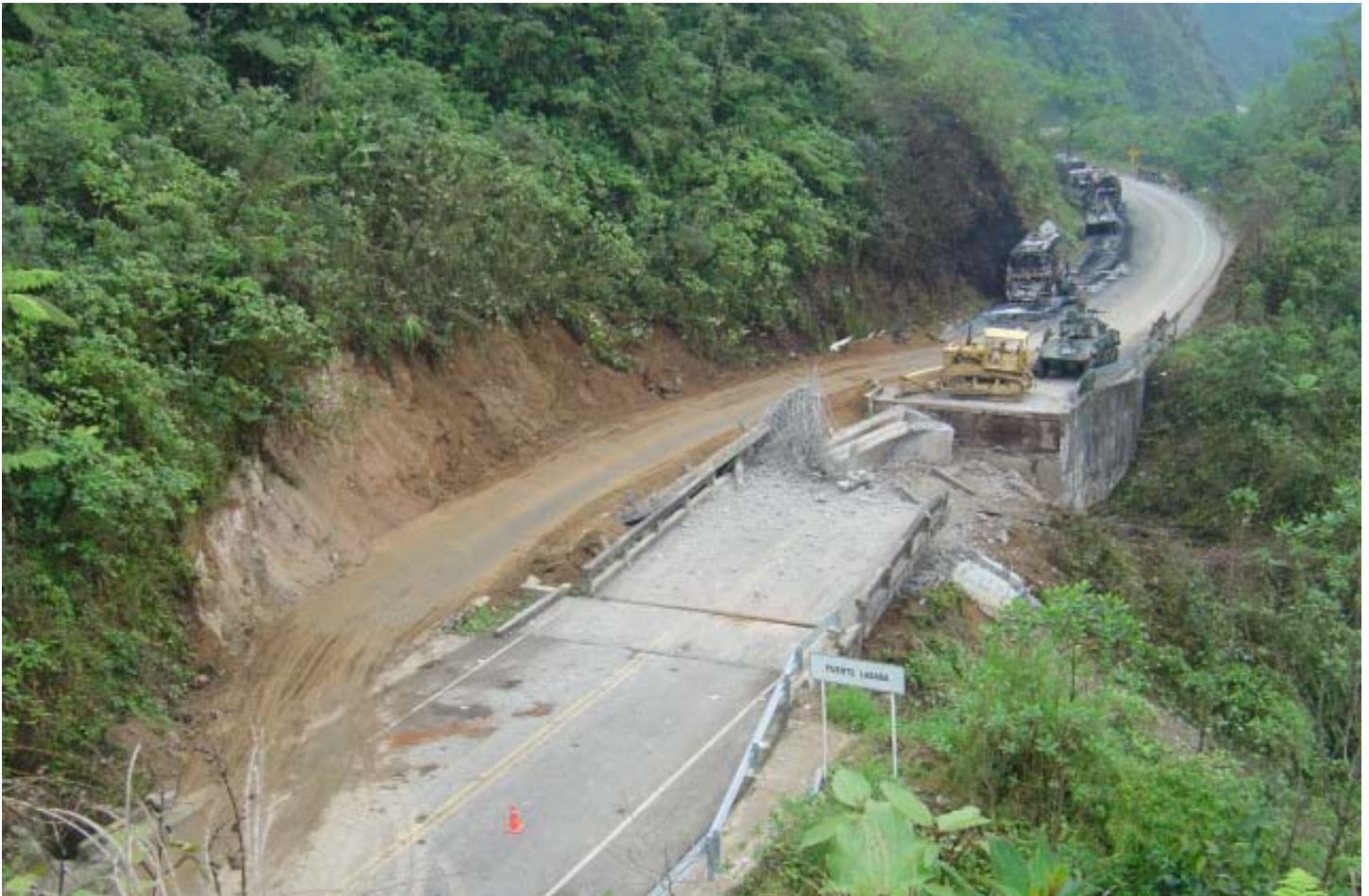
▲ ROADBLOCK An explosion on a bus caused by insurgents damages the road and inhibits travel. All photos provided by Patrick J. Christian.
