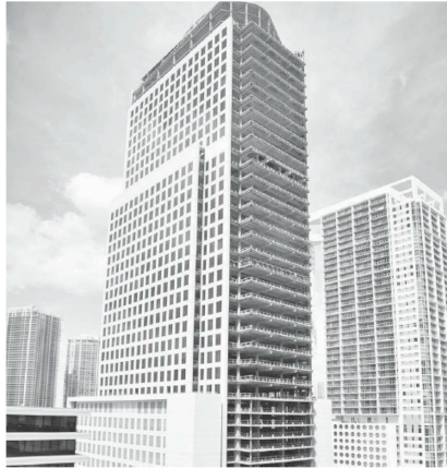
French bank is taking 20,137 square feet on 37th floor of 600 Brickell at Brickell World Plaza, shown in construction. A law firm is to follow.
