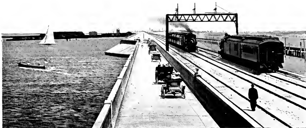
View of the Famous Causeway. Built of Reinforced Concrete. Is Two and One-Half Miles Long. Cost $2,000,000.
