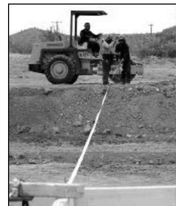
Brown & Root workers measure out ground for Camp America North and drive in a stake to mark the spot.
