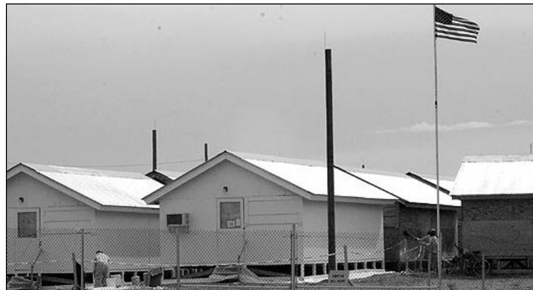
Two SEAhuts with a new coat of white paint (white will help reflect sunlight and keep the SEAhuts cooler) stand out from the yet-to-be-painted camp commandant's hut at the front edge of Camp America.
