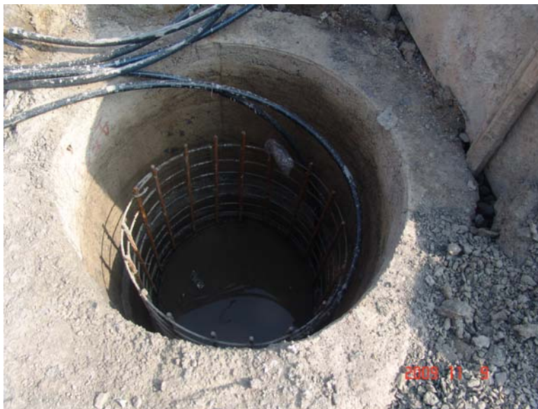
结构设置钢筋笼 steel reinforcement cage
