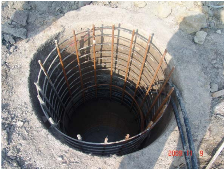
挖孔桩浇筑完成、初步成型 Drilled pile pouring the completion of the initial shape
