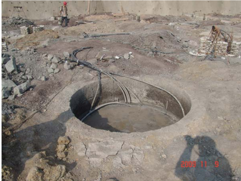
干管将各盘管连接形成换热环路 Main pipe will be connected to form each coil loop heat exchanger
