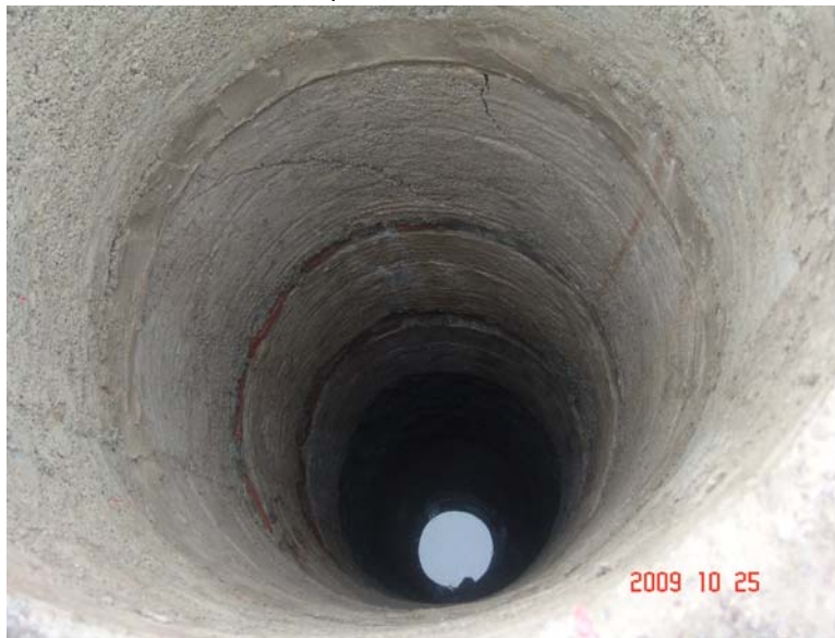
孔桩盘管施工过程 Pile coil construction process
