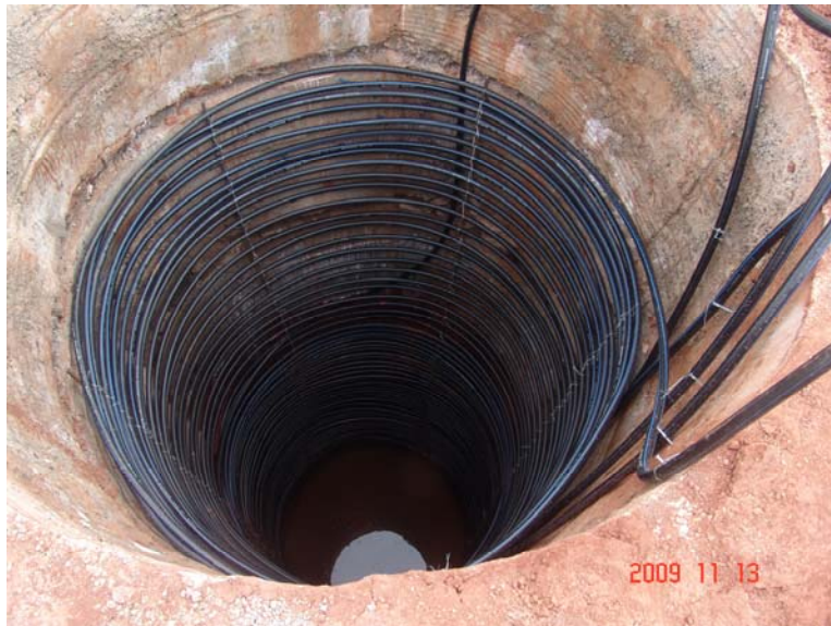
6 米深盘管施工成型 Construction of the 6 m deep coil forming
