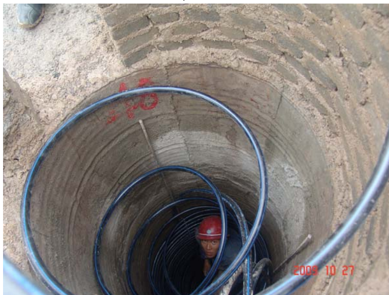
孔桩盘管施工完成 Pile coil construction completed
