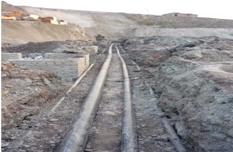
干管将各盘管连接形成换热环路 Main pipe will be connected to form each coil loop heat exchanger
