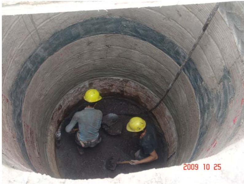
孔桩施工完成 Pile Construction completed
