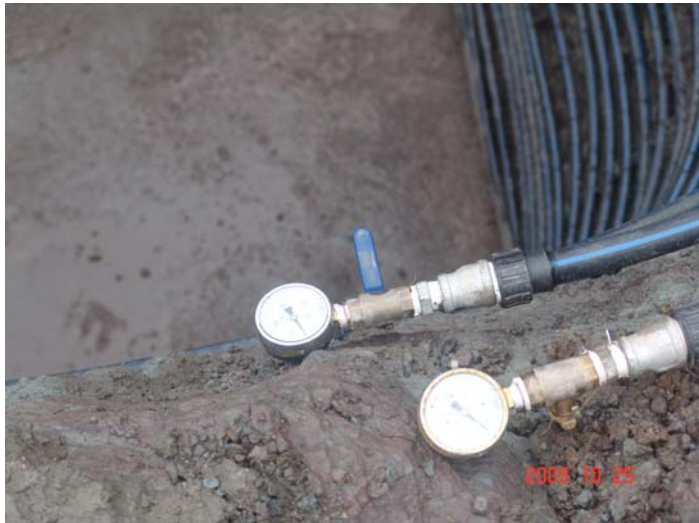
试压完毕、等待浇筑 Pressure test is completed, wait for pouring
