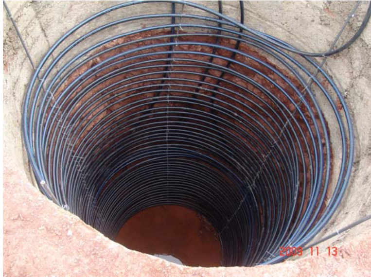
6 米深盘管施工成型 Construction of the 6 m deep coil forming
