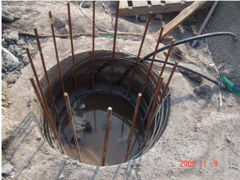
挖孔桩浇筑完成、初步成型 Drilled pile pouring the completion of the initial shape
