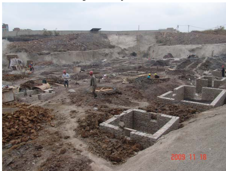
工地局部场景 The scene of building site in a part
