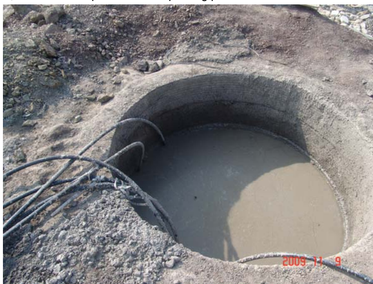
换热桩浇筑完成 The completion of heat pouring pile
