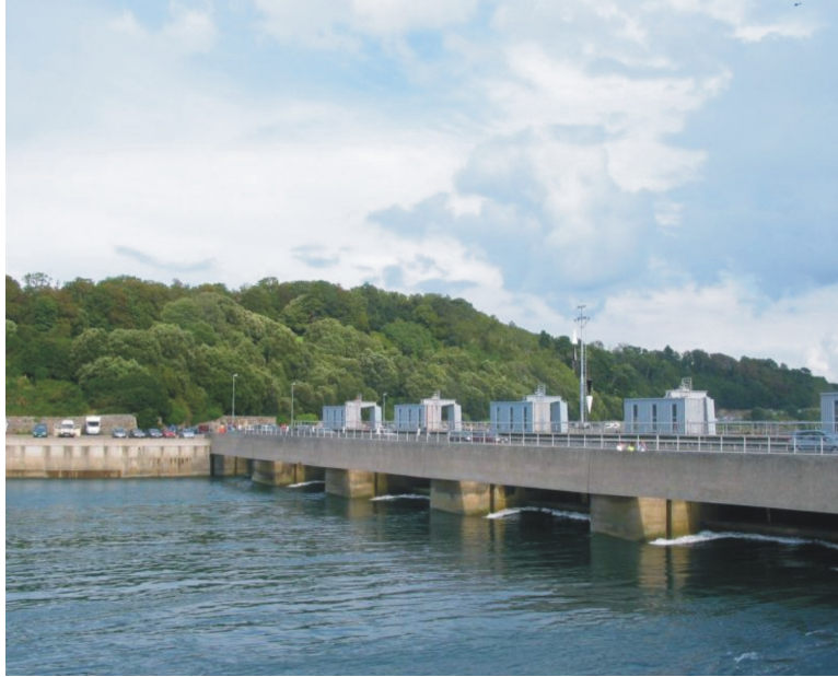
Figure 25.20: Dam of the tidal power plant on the estuary of the Rance River, Bretagne, France (37)
