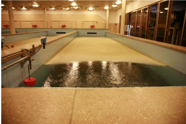
Figure 25.12: A water purification system at Bret Lake, Switzerland. Contaminants are removed and clean new water is created. (32)
