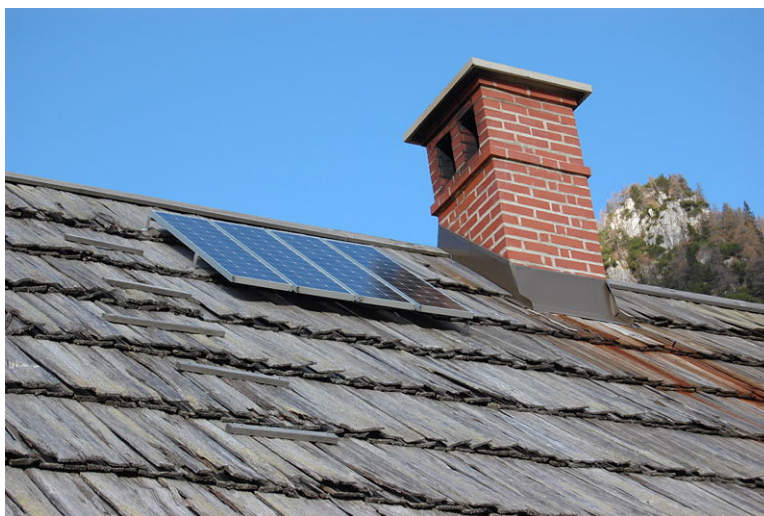
Figure 25.18: An example of solar power, using solar cells to convert sunlight into electricity. (16)
