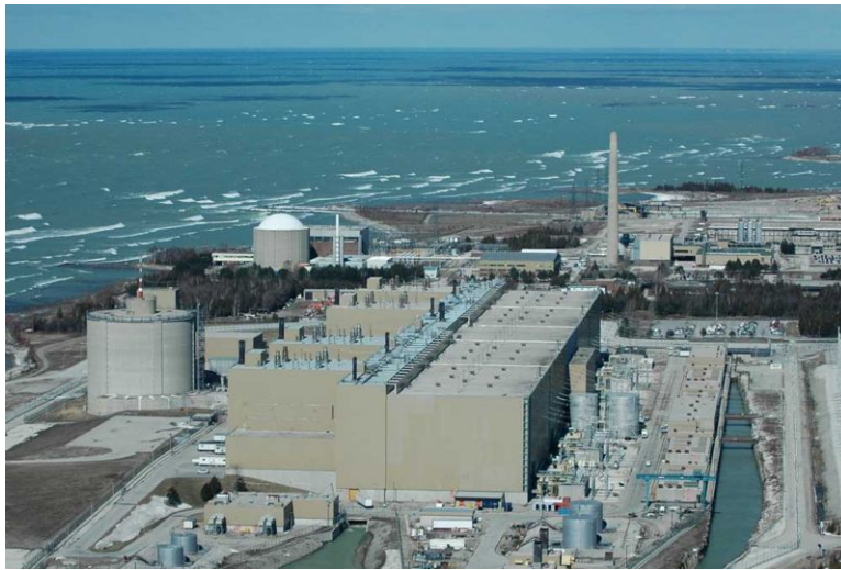
Figure 25.21: Aerial photo of the Bruce Nuclear Generating Station near Kincardine, Ontario (15)
