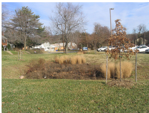
Figure 25.11: Intercepting nonpoint pollution between the source and waterway has been found to be successful. Pictured here, a bioretention cell, or rain garden, in the U.S, is designed to treat polluted storm water runoff from an adjacent parking lot. (4)
