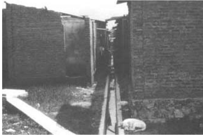
A surface water drain in Colombo, Sri Lanka. Although the area is crowded, the drain is kept reasonably clear as it passes through the front yards of the houses.
