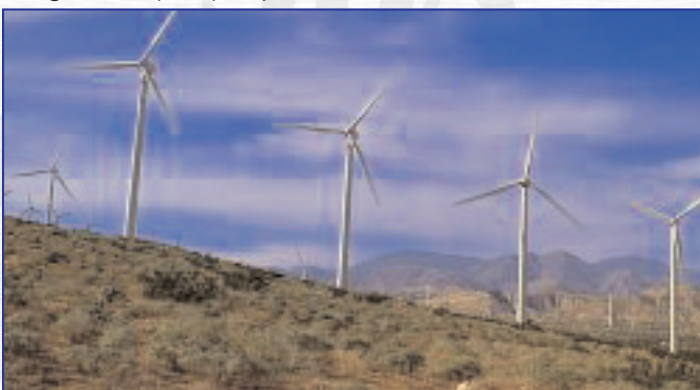
A section of the Wigton Wind Farm - Manchester.
