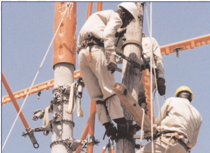
JPS Linemen working together as a team.
