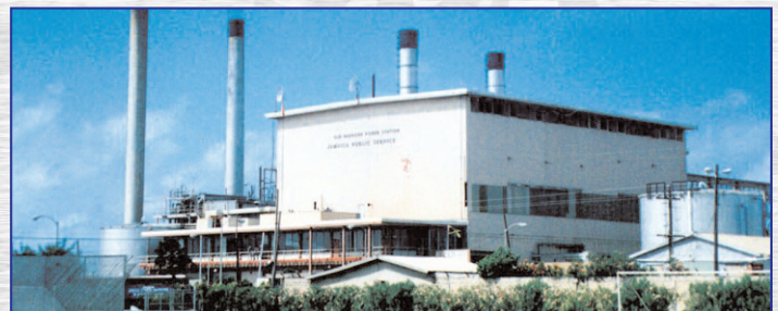
Hunts Bay Power Station in Kingston
