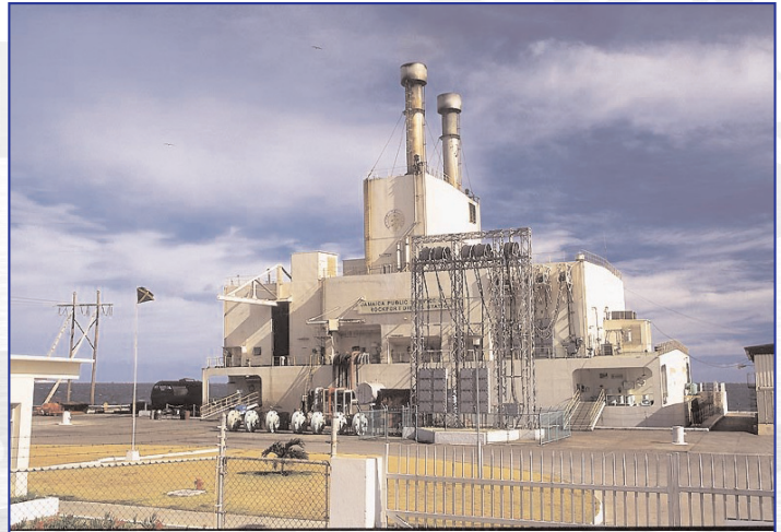
Rockfort Power Station.
