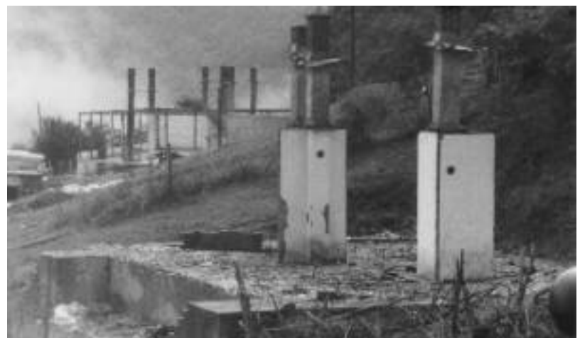
Destroyed school in Kotlina [zoom]
