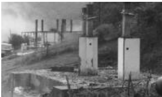
Destroyed school in Kotlina [ zoom | reference ]
