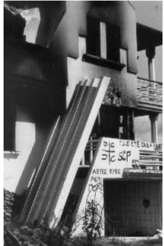
Kosovska Mitrovica: a looted and burnt out house in the hospital district. The graffiti read: "Where are you now Siptars", "Pretty house pretty flame" and "Serbs don't protect Siptars"
