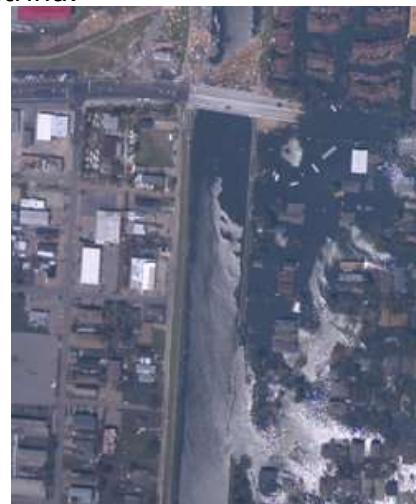
Closeup of 17th Street Canal breach in New Orleans
