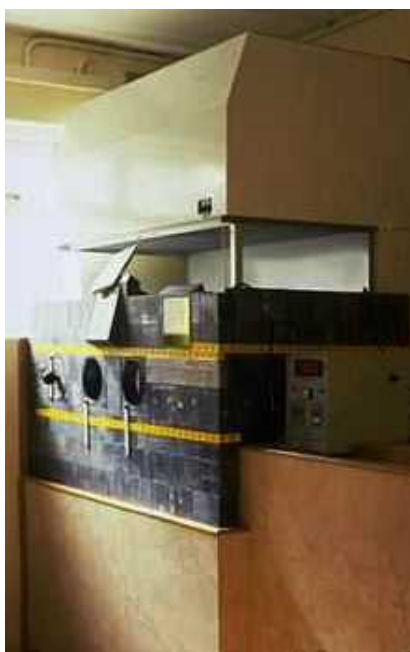
Pb shielding surrounding the laminar flow cabinet, where radiopharmaceuticals are prepared.
