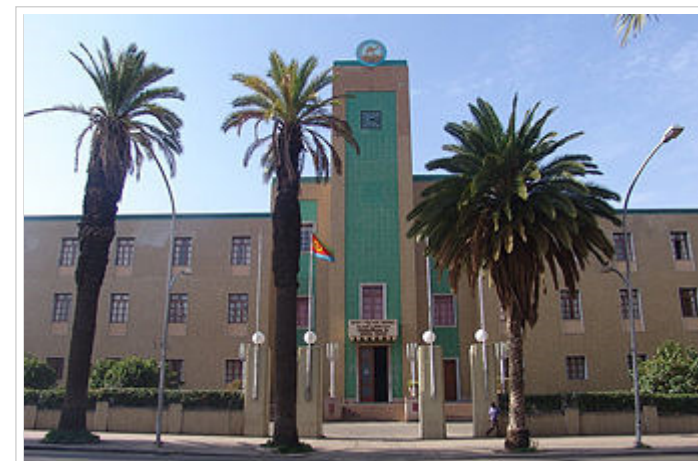
Government building of Eritrea in Asmara
