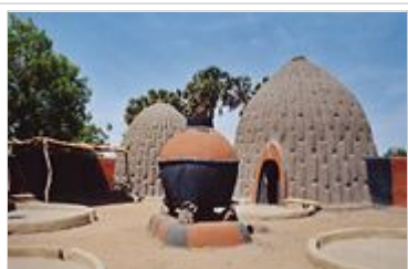
The homes of the Musgum, in the Far North Province, are made of earth and grass.
