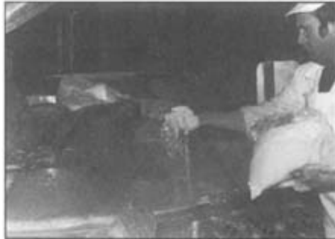
141. Improper handling: dosage by hand
