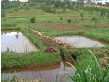
Poorly constructed earthen ponds
