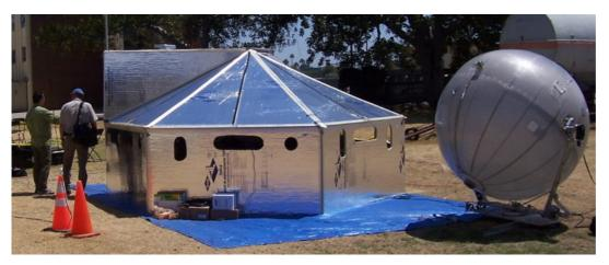
This Hexayurt was made from about \$200 of materials, mostly from Home Depot, and took three hours from unloading the truck to a finished building. The ball is an inflatable T1 to orbit (http://youtube.com/watch?v=DomTyuxiSbQ).
