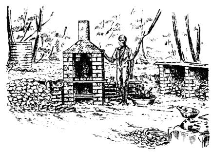
A kiln for small-scale firing trials.
