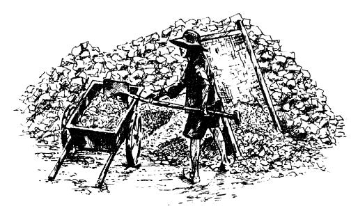
Using a coarse sieve for low grade dry hydrate.
