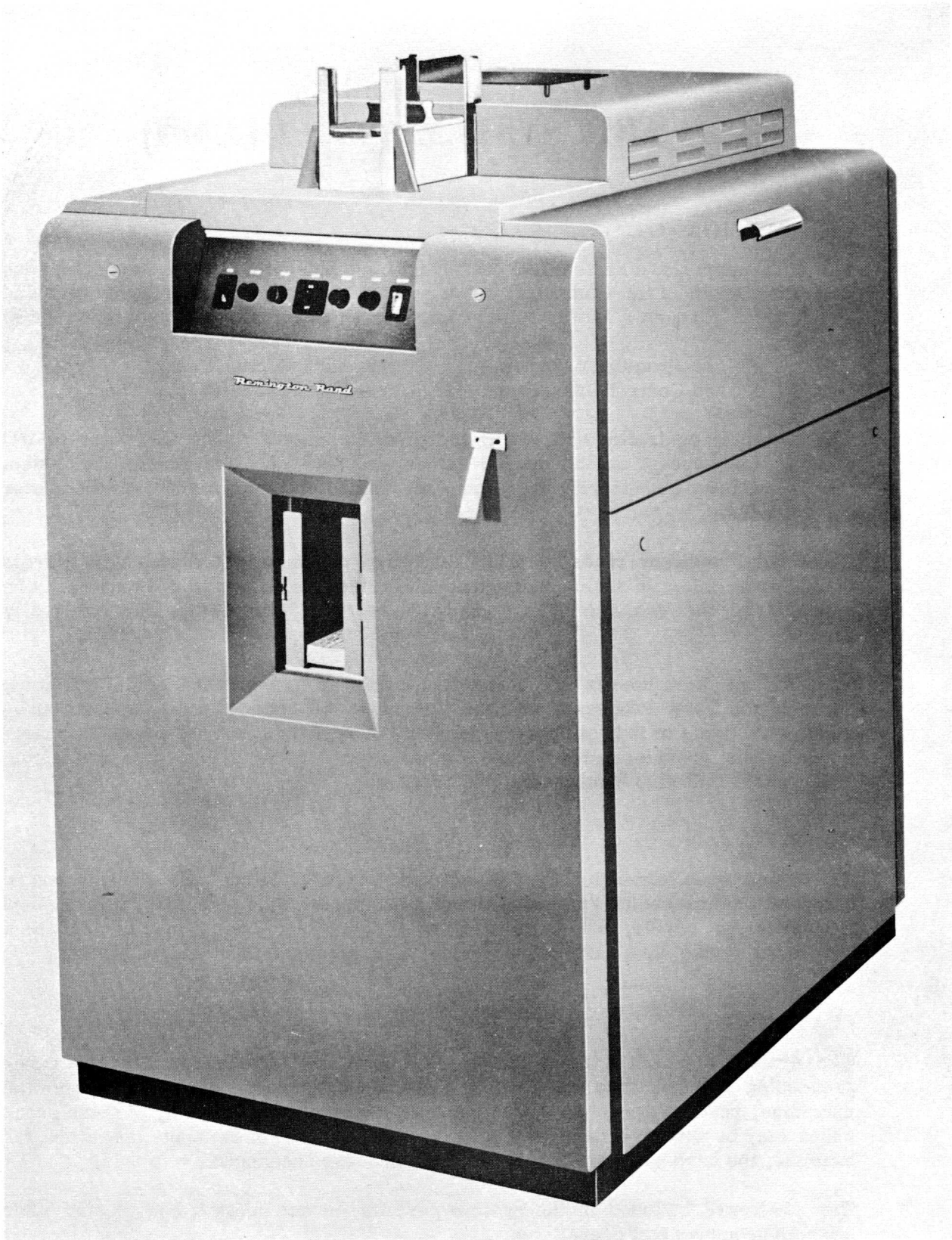
Card-to-Paper Tape Converter
