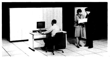
Amdahl, the original PCM supplier, offers two IBM-compatible computer families: the 470 Series and the 580 Series. The 580 Series was announced in November 1980 as a replacement for IBM's 3081 processor. The 580 Series consists of the single-processor 5860 (shown here) and the dual-processor 5870 and 5880. The 580 Series processors feature from 16 to 32 megabytes of main memory and from 16 to 34 I/O channels per CPU.
