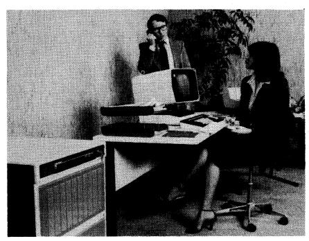
ICL's System 25 includes a cabinet that contains multiple microprocessors, a Winchester disk drive, and tape cartridges for software exchange. Also shown is a Model 3485 visual display unit, one of several workstations available, and, in the background, a 180 cps printer.
