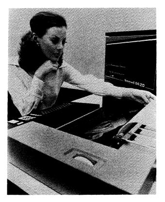
The Model 64/20 features optional microprogrammed emulation of the Honeywell Series 200/2000 and Series 100 systems and is considered the logical upgrade system for most of the current small-scale installations in Honeywell's large customer base. System rental prices range from approximately \$5,000 to \$10,000 per month.
