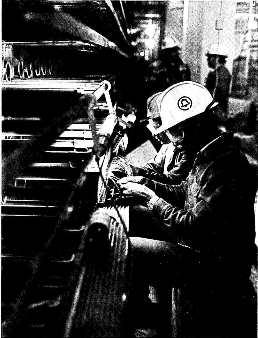
The intricate job of wiring proceeded day and night on the new main distributing frame in New York Telephone's burned switching center. Shown are two Western Electric installers.
