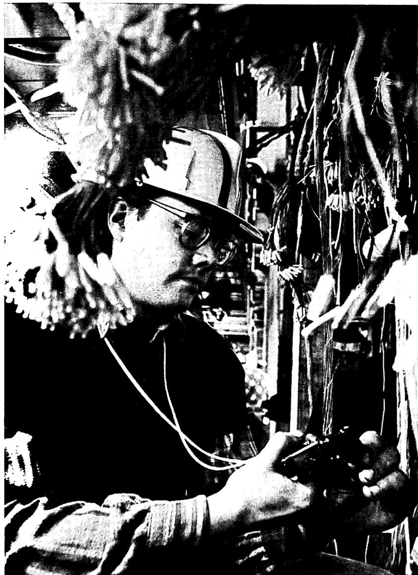
New wires dropped from overhead cable and ready to be connected have the attention of this WE installer. He's one of the approximately 1,200 WE installers who were on round-the-clock duty in the aftermath of New York Telephone's terrible fire.
