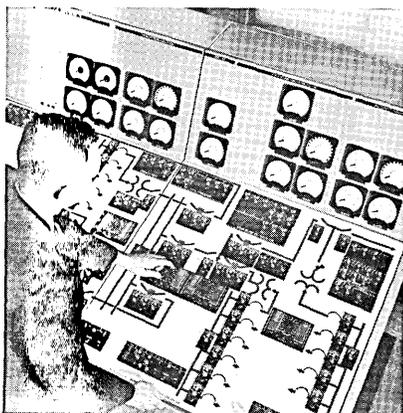
— Operator at the control panel (shown above) of the new SUPER-TROL II Control System receives status reports from each remote station every 24/1000th of a second
