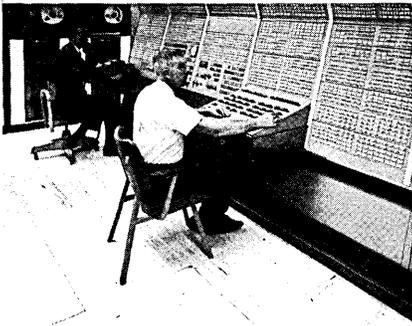
— Data Processing Central (DPC), Project 465L, Prototype Equipment located at the ITT Data and Information Systems Division test facility.
