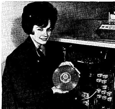
— NCR 395 magnetic disc memory is shown here in front of some of the system's 250 logic modules.
