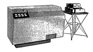
The RW-300 Digital Control Computer is the most powerful tool available today to control entire industrial processes and to provide useful data from manufacturing and testing operations. Connected directly to measuring instruments and control devices, the RW-300 collects and interprets operating data, makes control calculations and decisions, and operates valves, starts and stops motors, and takes all the other control actions necessary for fully automatic operation.
