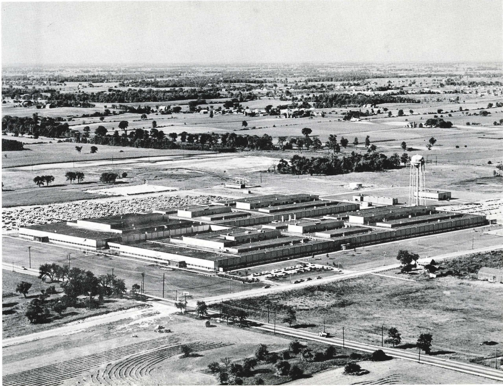
Figure 8-1. AC Spark Plug Division — Milwaukee Oak Creek Facility
