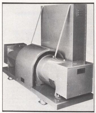
Rotary motor generators such as this Atlas unit come with power cables and are about one-third to one-half the cost of static UPSs. They have a 5- to 750-kVA rating and are housed in a soundproof, weatherproof enclosure.
