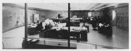
**Technicians monitor and control power flow** through 325 substations form Con Ed's Energy Control Center.
