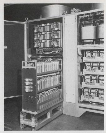
Massive power source on wheels: one of three Teledyne Inet inverter switching sections, mounted on rollers for maintenance convenience.
