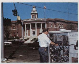
This traffic controller is a key element in a Connecticut system by Automatic Signal, Norwalk, that cut travel time by 45% through a high-traffic shopping district. Local intersection control is exercised by a CMOS microcomputer that talks to the system computer.
