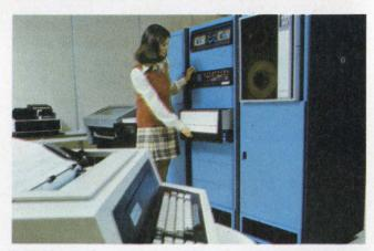
A 32-bit minicomputer with 1 Mbyte of core cycles at 450 ns average, 300 ns minimum. Interdata's 8/32 Megamini uses high-speed Schottky-TTL circuits.
