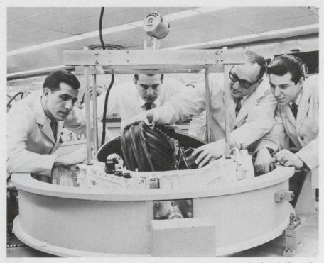
**Three control-moment gyros,** like this one, control the attitude of the telescope mount within  $\pm 2$  minutes of arc. Each gyro is 22 inches in diameter and spins at about 9000 rpm. For backup, conventional gas nozzles are used.
