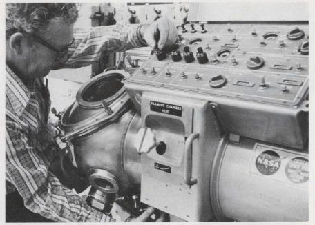
**Manufacturing facility** in Skylab consists of a vacuum work chamber 16 inches in diameter with four-inch-diameter opening to space. Tests will include electron-beam welding, crystal growing and metals melting.
