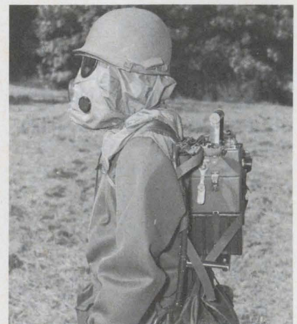
M8 chemical alarm system can detect minute amounts of nerve gas.
