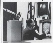
An infrared light beam carries data between an IBM System/360 computer in the Canadian Government pavilion at Expo 67 and a receiving unit and graphic display terminal (above) in the Man the Producer pavilion half a mile away. The path of the beam has been simulated by photographic retouching. Polarad modular microwave signal instruments offer you new flexibility. Build the system you need now, rearrange or add new modules later.
