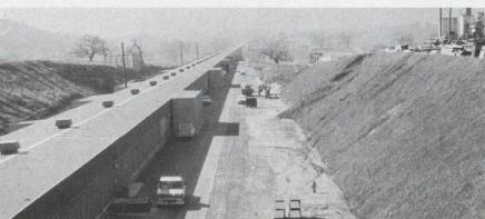
SLAC comprises two main elements, both extending over the 2-mile length. The accelerator housing (left) is an 11-foot-wide by 10-foot-high underground tunnel that contains the accelerator proper and related systems. The klystron gallery (right) is a 29-foot-wide by 13-foot-high above-ground installation containing the klystrons, modulators, vacuum pumps and other auxiliary equipment.
