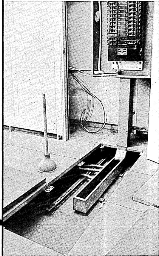
*Electrical power panel entry into floating floor.*
