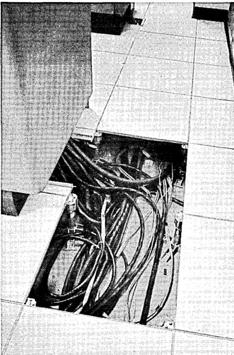
*Floating floor panel makes it easy to feed air directly into machine.*
