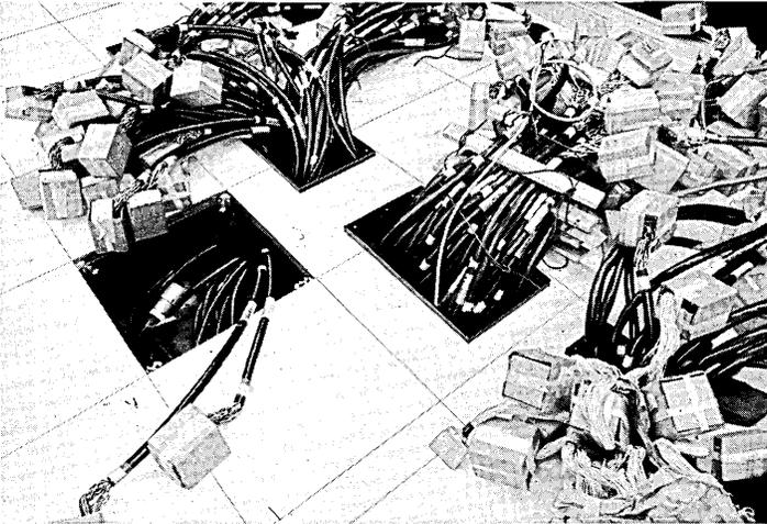
*Unusual conditions can be met with floating floors. Cable cutouts can be located at any place required. The raised edges prevent casters from dropping into cable opening when moving machines.*
