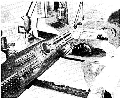
Yardmaster W.L. Timmons directs the operation from his office high above the tracks. The cars are lined up in front of a switch engine that slowly pushes them to the crest of a man-made hill some 35 feet high. Just as they reach the top, they are uncoupled and start to coast down the other side of
