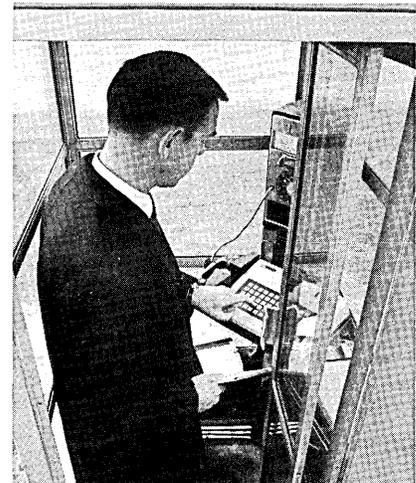
The handset of the telephone fits into the terminal's acoustic coupler, which transmits the user's signals; the computer's reply is heard over the terminal's built-in speaker, or through an earphone. The IBM 2721 has 60 keys, 26 letters, 10 numerals and 24 special characters and controls. These can be adapted for specific applications with the use of plastic keyboard overlays. To prevent unauthorized access to data stored in the computer, each 2721 can be assigned an identification code.
