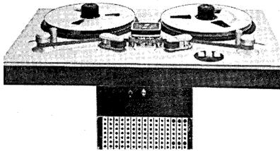
The G-12, because of modular design, can be matched for any combination of up to 20 duplicating slave recorders and can be patched in or out of the common bus without system readjustment. Two, four or eight track magnetic heads may be plugged in quickly to handle a wide variety of program formats.
