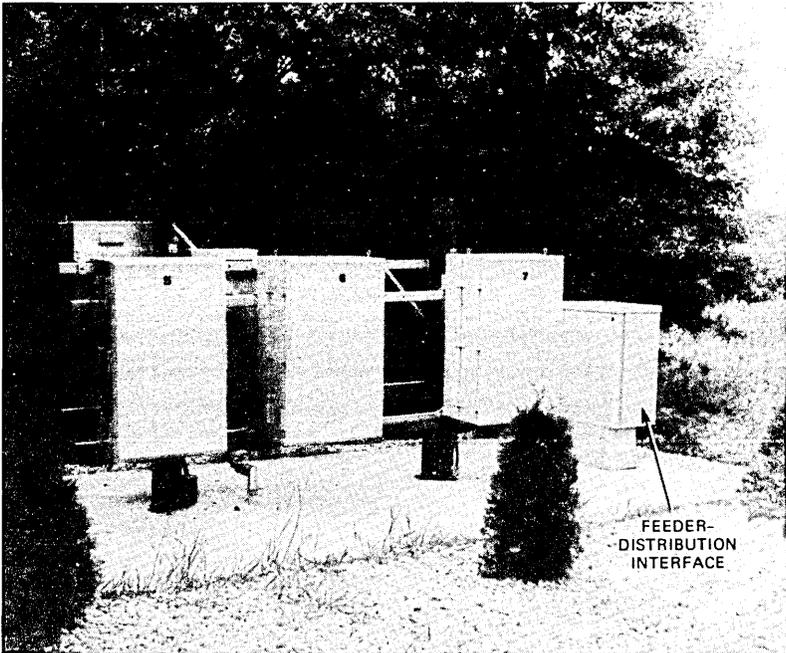
Fig. 11—Configuration of 36-type cabinets mounted on crossarms.
