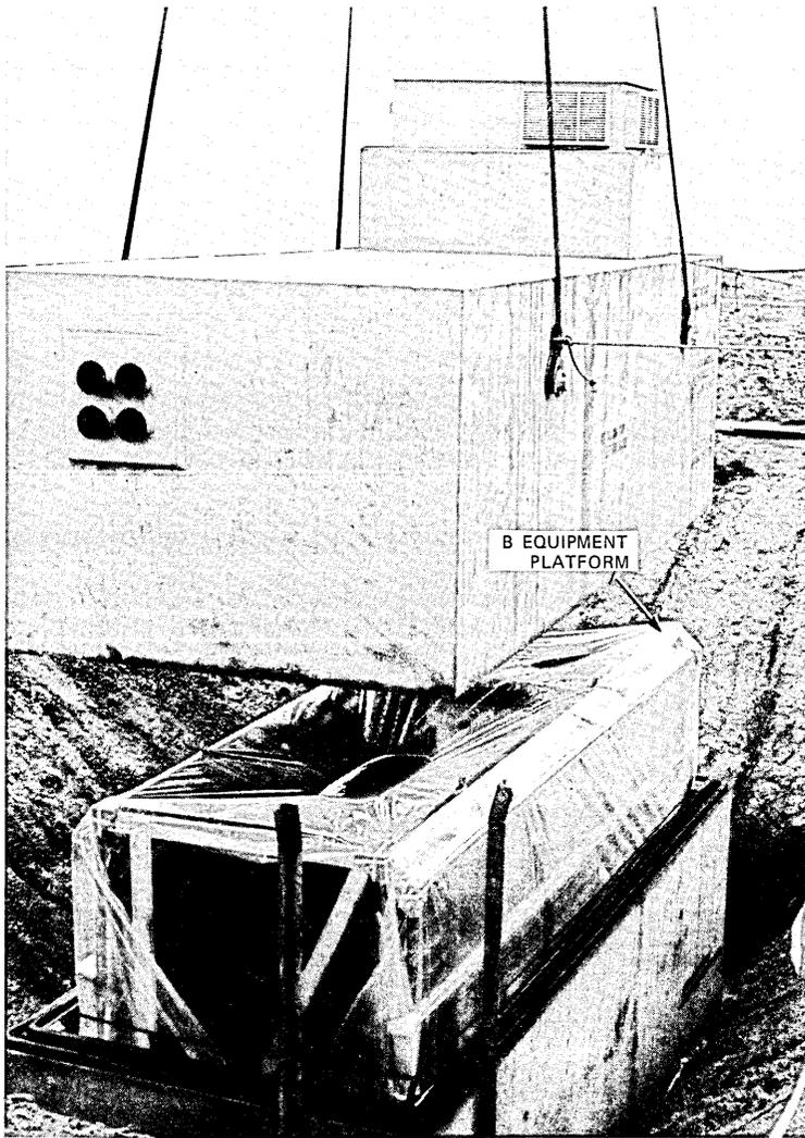
Fig. 20—Placement of a controlled environment vault with a B equipment platform.
