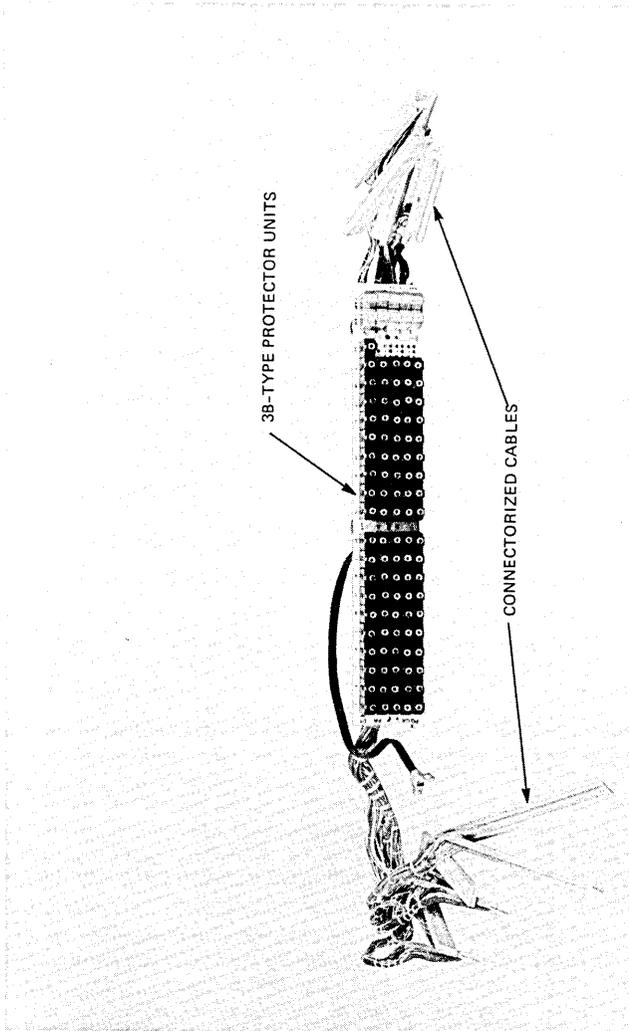
Fig. 8—Bank-mounted protector assembly.
